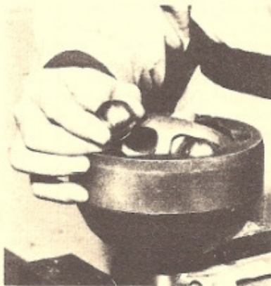
Figure 114 — Tilting inner race.
